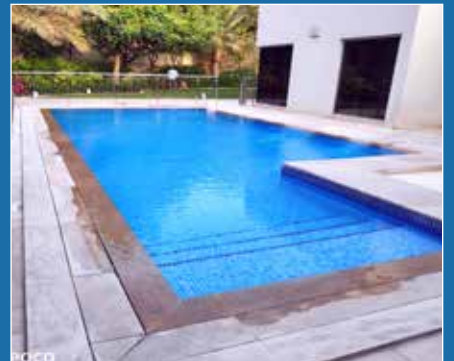
Overflow Pool, Al Khawaneej
